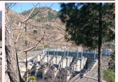
A view of the Pandoh Dam.
